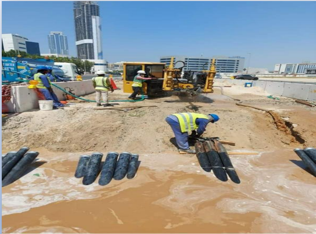
Horizontal Directional Drilling(HDD) for DEWA 132KV
