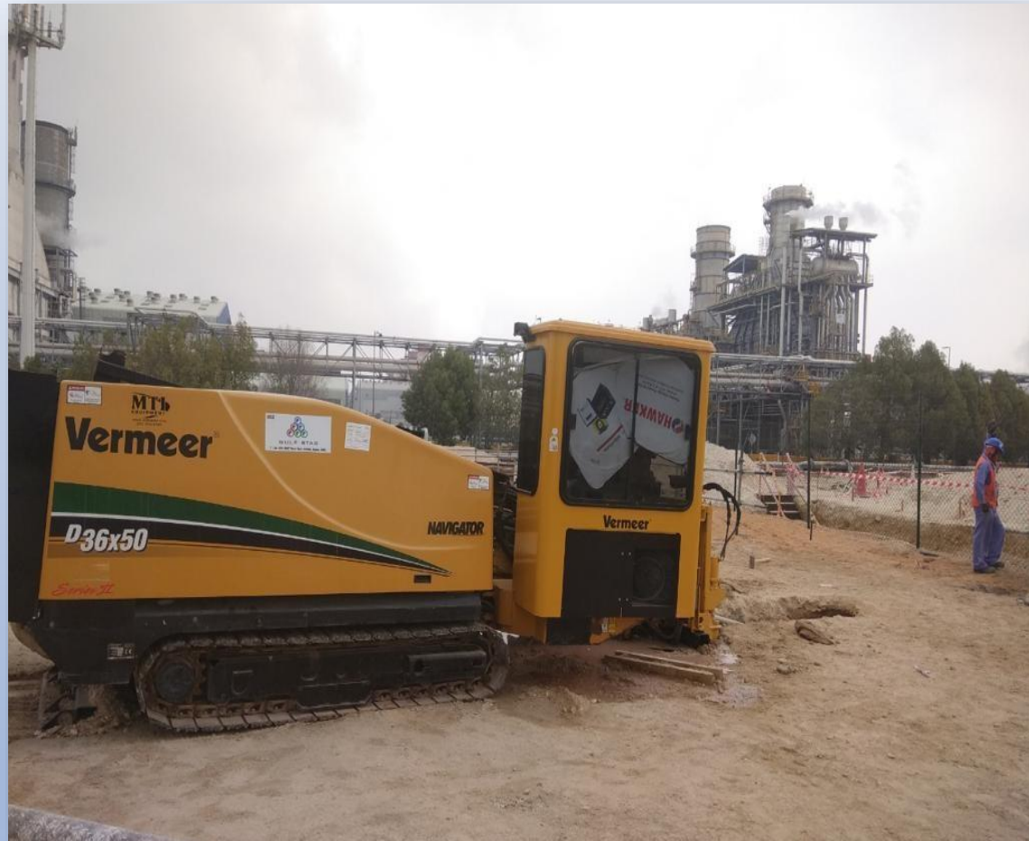
Horizontal Directional Drilling(HDD) for DEWA Scada Works
